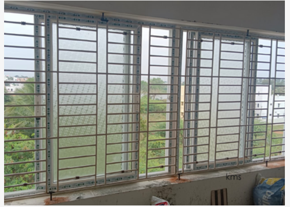
WINDOWS & GRILL WORKS
