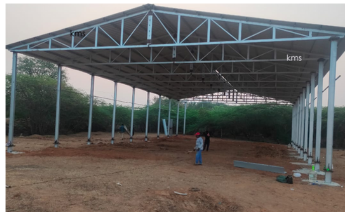
METAL ROOFING SHEDS
