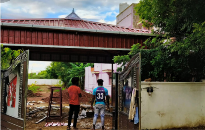
KERALA ROOFING SHED
