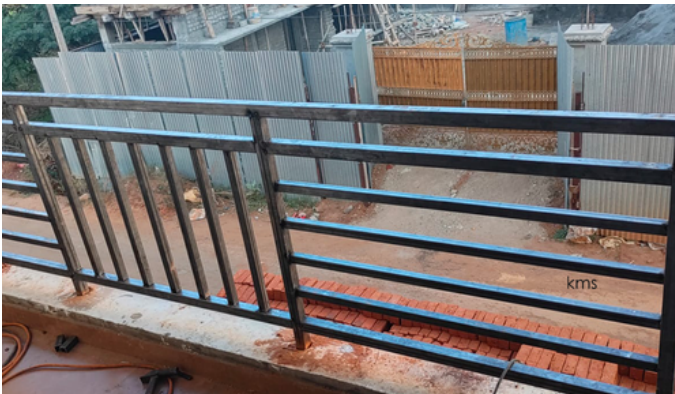
MS BALCONY RAILING
