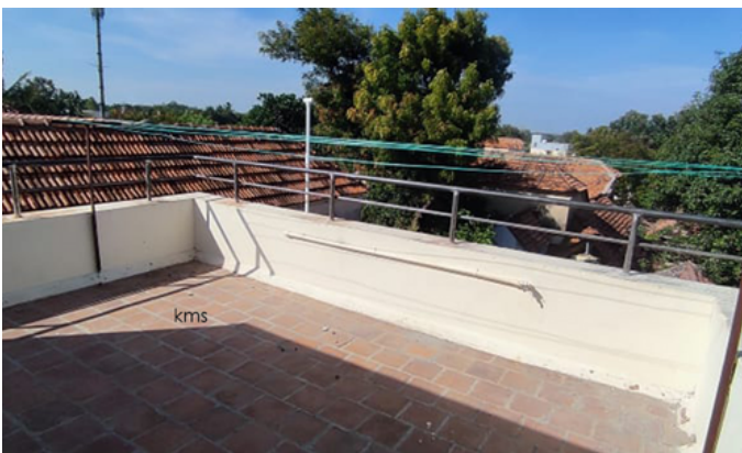
STAINLESS STEEL BALCONY RAILING
