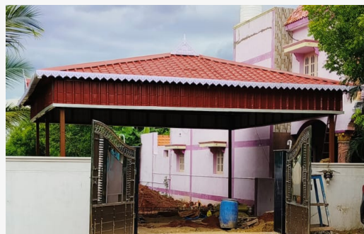
ROOFING STRUCTURAL WORKS
